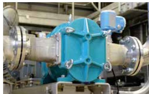
BLUEline pump for conveying cleaning agent
