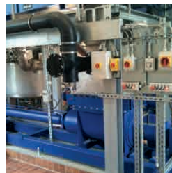
Conveyance of sludge from decanter to silo: KL65RÜ80.4 ESP with fill level monitoring
